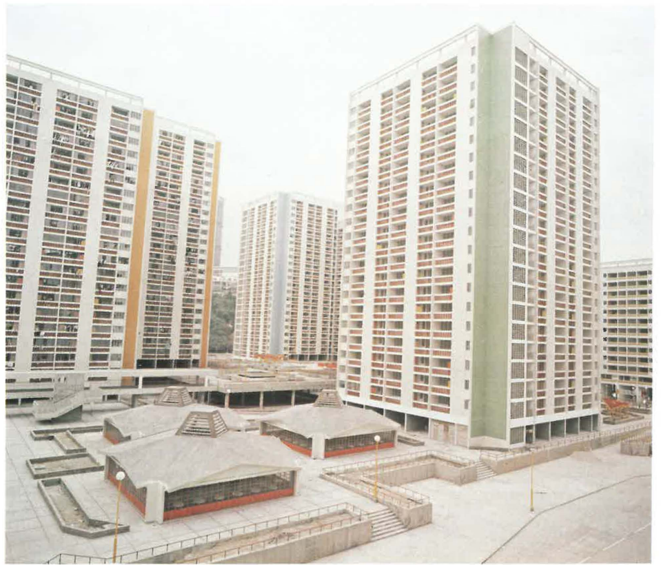
While Government rented accommodation continually evolves better standards : Wo Che Estate at Sha Tin
